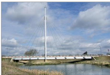
Fig D - Broughton cable stay bridge
